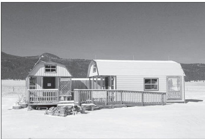
Old temporary visitor center
