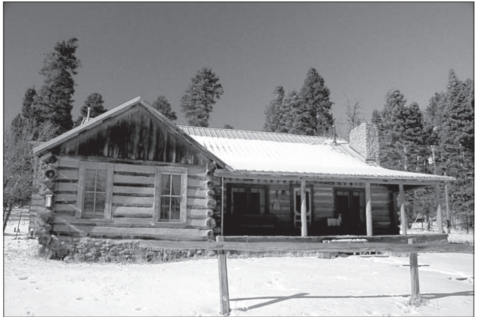
Figure 4: Original Baca Ranch Owner's Home
